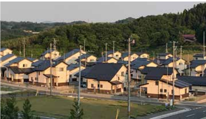
Restoration public housing was constructed in Egenokoshi and Hirasawa districts in Miharu Town.
