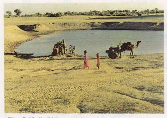
${f Fig.~7~Nadi}$  (Village tank) - A traditional rainwater harvesting system for domestic water supply and livestock consumption.
