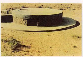
Fig. 9 An improved tanka of 21,000 litres developed by CAZRI.
