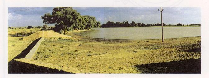
Fig. 8 Khadin - A traditional rainwater harvesting system for crop production.
