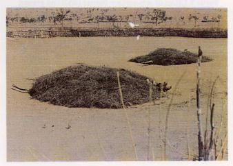
Fig. 6 Tanka(cistern) - A traditional rainwater harvesting system for drinking water.
